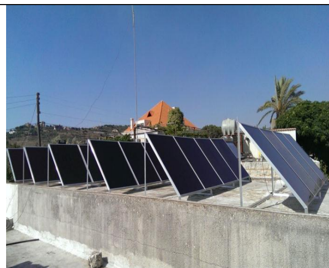
Qubeyeet centralized solar street lighting
