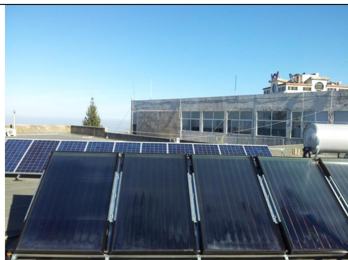
Aley Prison Dual SHW and PV system
