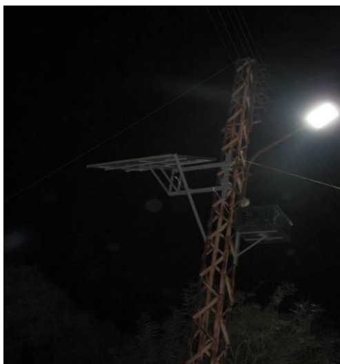
Roumin Street Lighting (PV system with LED lighting)
