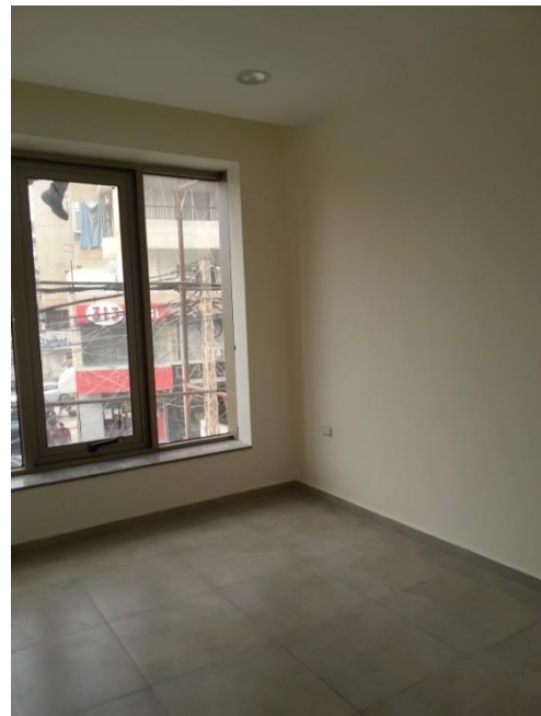
Painting and Tiling of the Rooms
