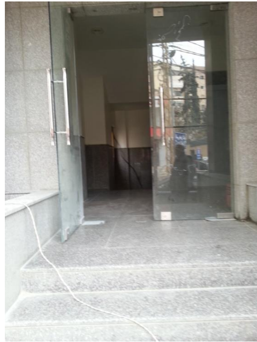
Granite Stairs and Cladding at the Entrance
