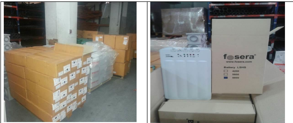
Contractor's warehouse ready for installation beginning May 2015
