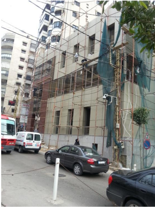
Curtain Walls installed on the external wall
