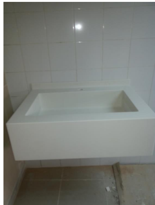
Medical Room Sink Installed
