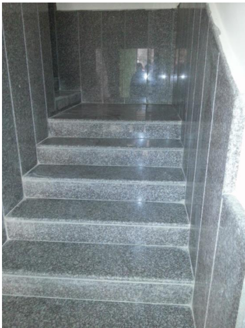
Staircase Granite Tiles
