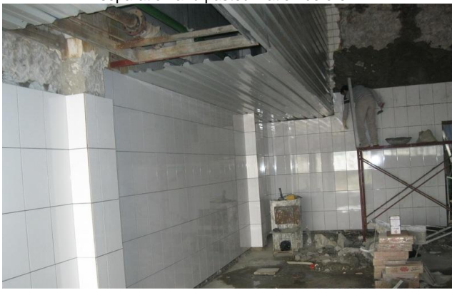
Civil works in progress
