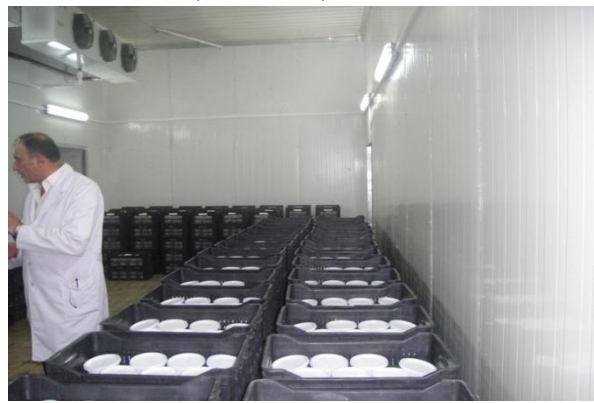
Rehabilitated cooling room
