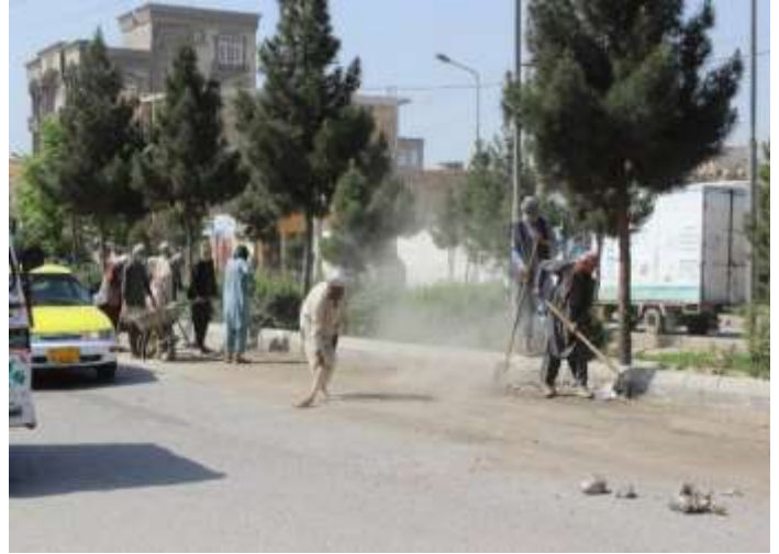
(During) Waste Disposal CFW Project in PD5, GA#11 of Mazar-i-Sharif
