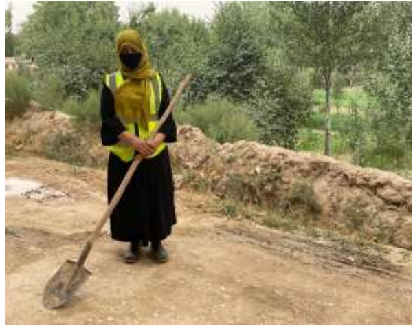
Young woman doing road maintenance in Aybak District (Sufihaa) (UNOPS/Constanza Malagamba)
