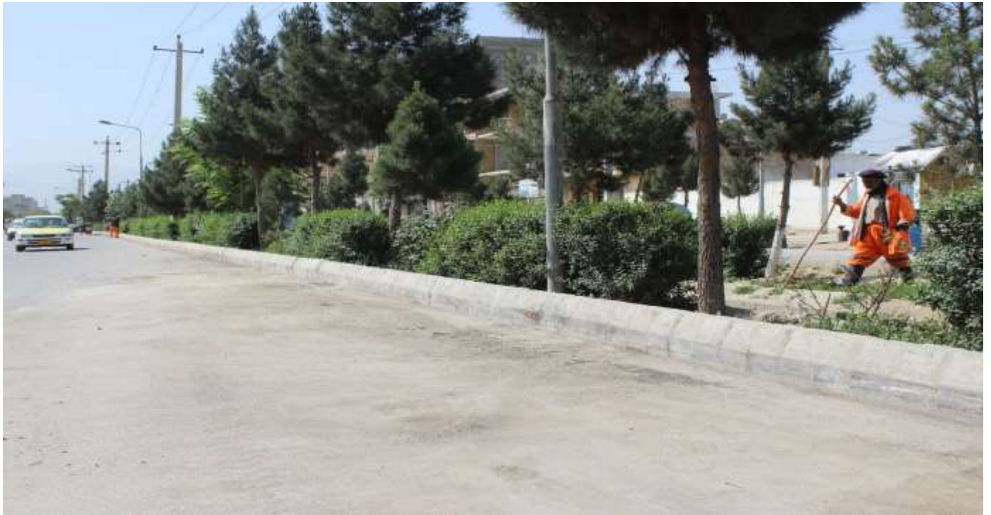
(After) Waste Disposal CFW Project in PD8, GA#1 of Mazar-i-Sharif
