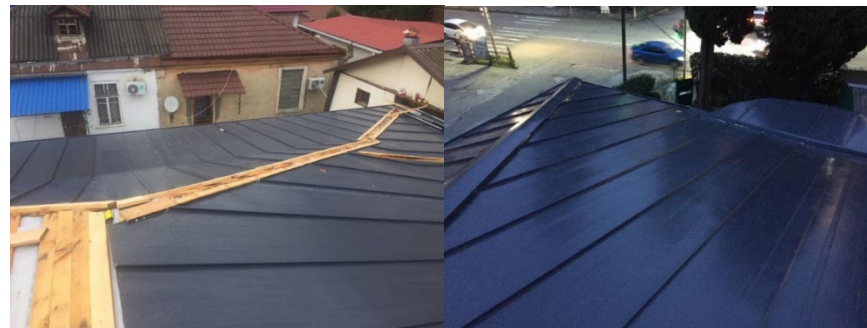
GMS roof rehabilitated
