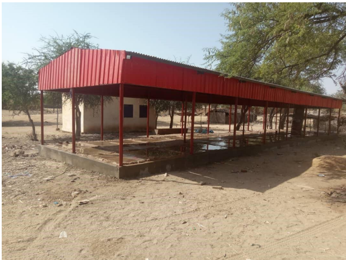
The market under construction (November 2021)
