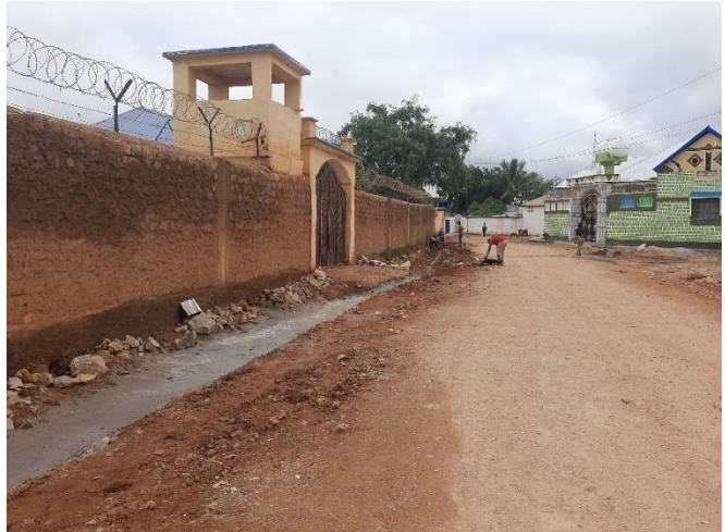
Maintenance of the road ©IOM Somalia
