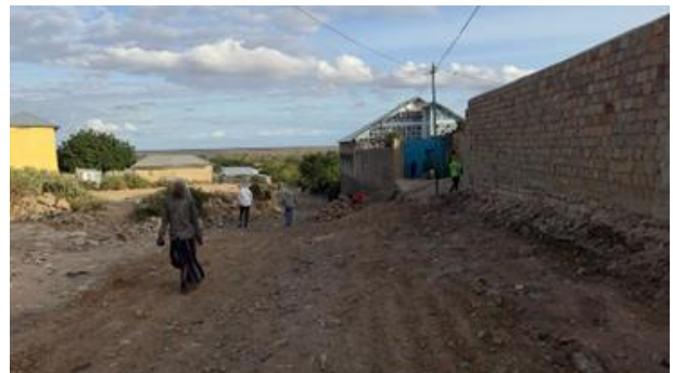
After maintenance of the road ©IOM Somalia
