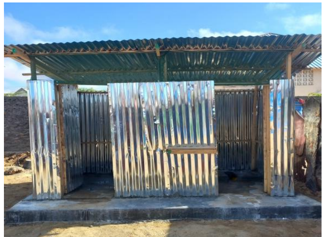
Constructed latrines ©IOM Somalia
