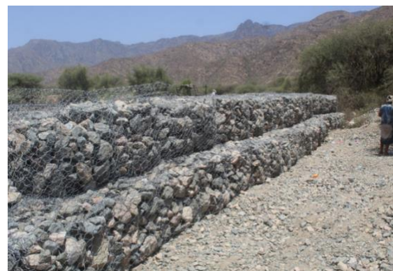
A constructed gabion wall in Lawdar, Abyan
