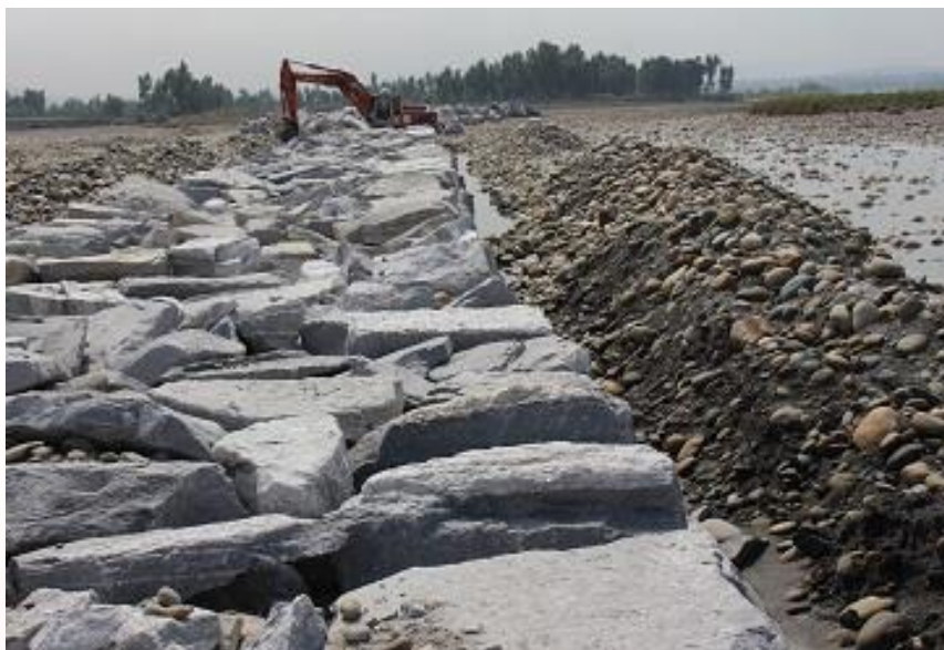
New Stone Boulder Wall constructed in Zakhil Kama Nangarhar, Eastern Region
