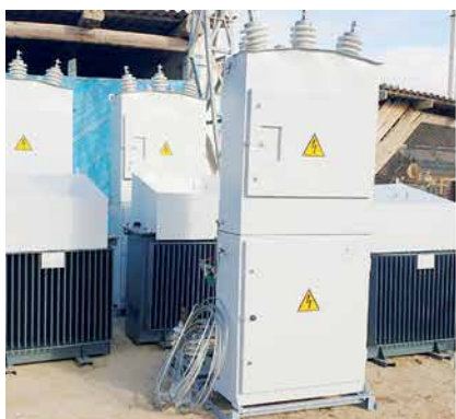
Photos 27, 28, 29: Transformers 250 kVA (17 communities) in Bozatau, Kungrad and Muynak districts.
