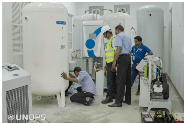
Installation of the oxygen plant
