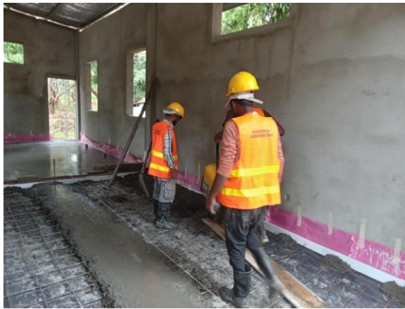
Construction of Plant Room in Kantale Base Hospital
