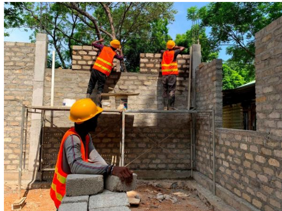
Construction of Plant Room in Mullaitivu DGH
