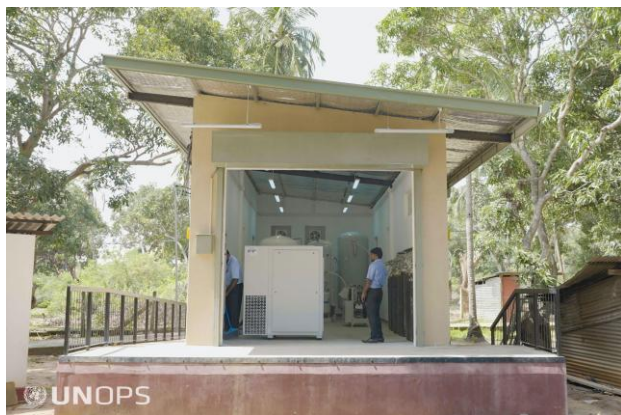
Plant room constructed under the project, Mullaitivu
