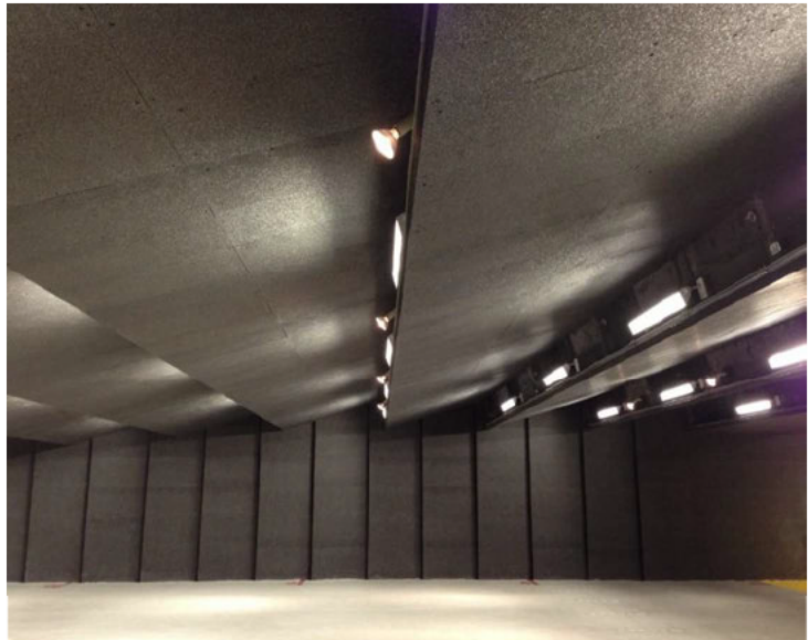
Figure 1. Example of safety baffles in an indoor shooting range
