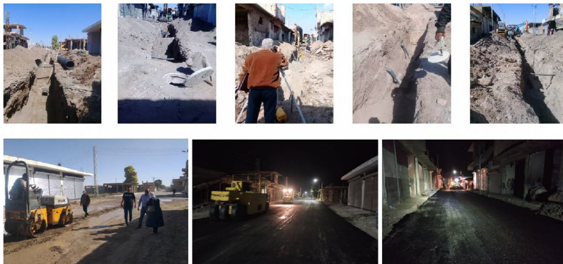
Figure 11, Rehabilitation works of sewage pipelines in the industrial area of Deir Ezzor City,
