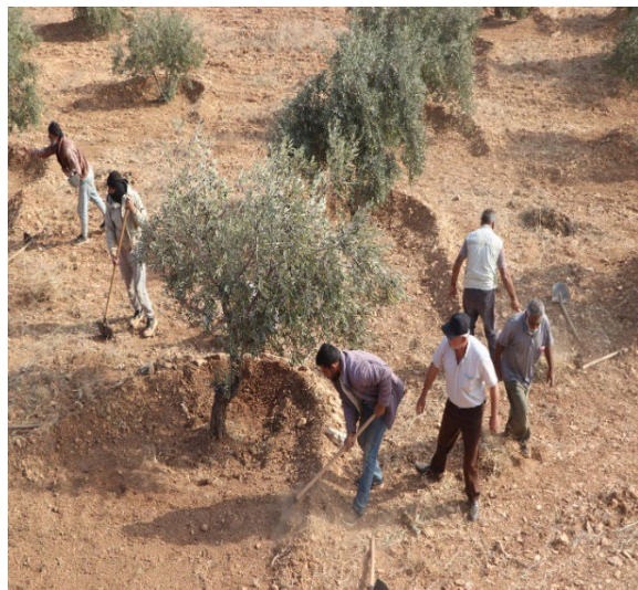
Figure 7- installation of rainwater harvesting bunds.
