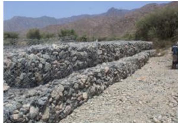
A constructed gabion wall in Lawdar, Abyan
