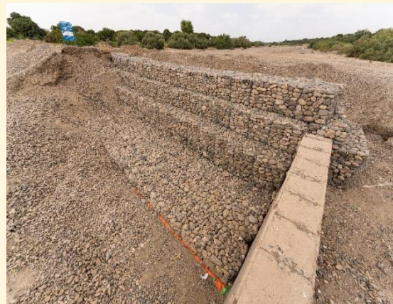
The gabion in Lahj prevents soil erosion and stores water, ensuring sustainable farming under the ERRY III Joint Programme.
