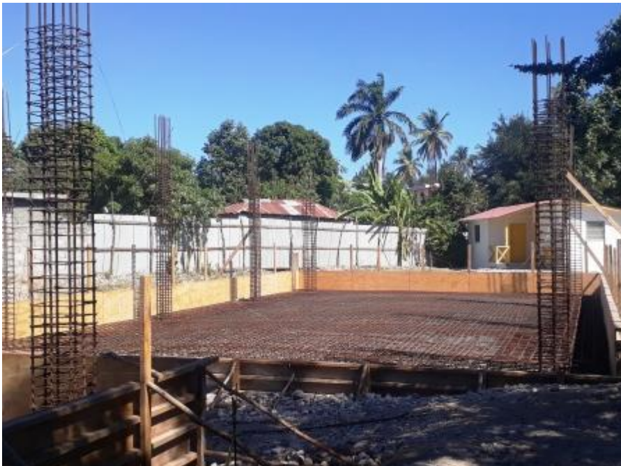
Finished reinforcement awaiting the pouring of concrete
