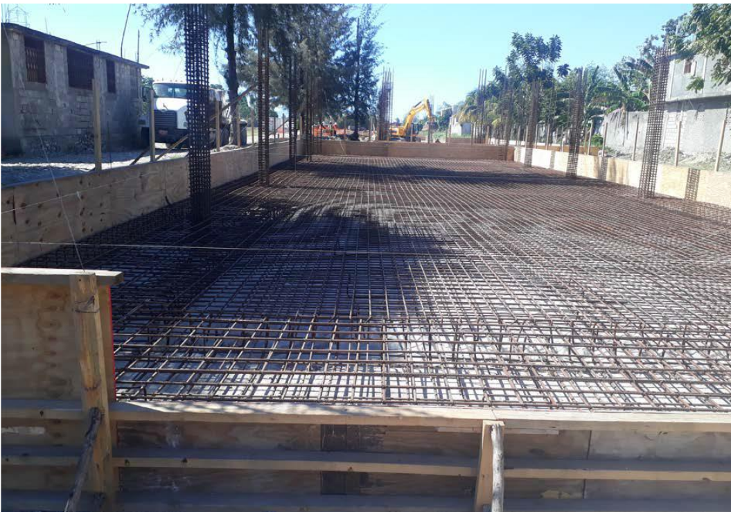
Finished reinforcement awaiting the pouring of concrete
