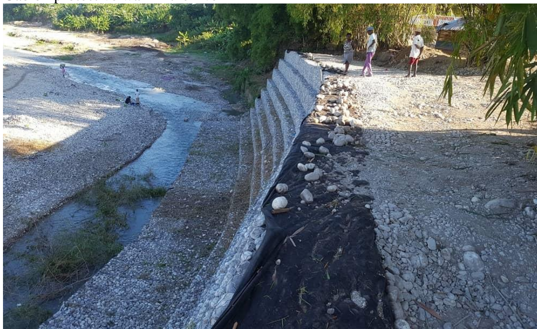
Gabion protective wall in the river
