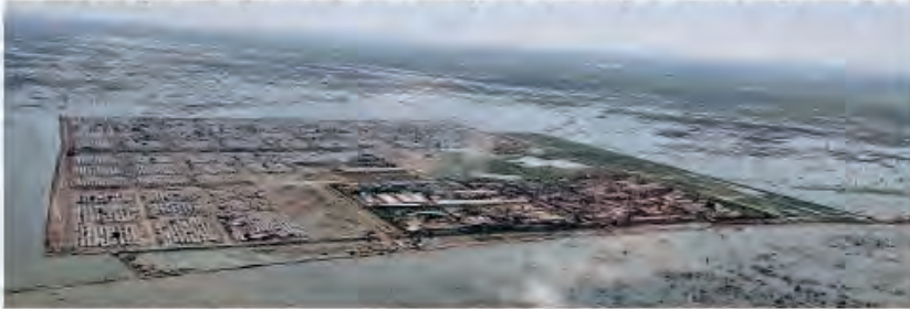
Figure 5: BOA: Bentiu Field Office
