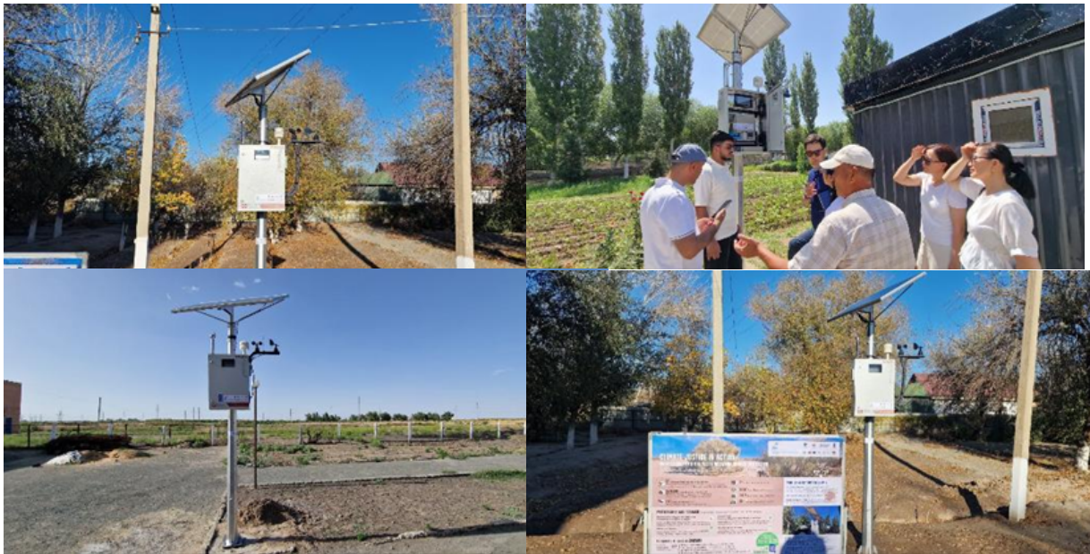
Photos 60,61,62,63: Established AQMS equipment in Karakalpakstan
