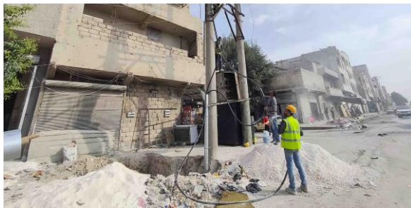
Figure 2- Electricity poles rehabilitation in Qadi Askar
