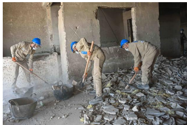
Figure 4- Debris collection and removal.
