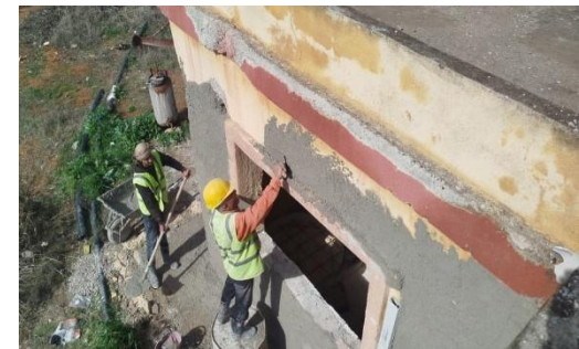
Figure 18- rehabilitation work for the management centre of Al-Safira irrigation project.
