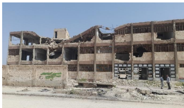
Figure 7- Husein Ibrahim – School Rehabilitation
