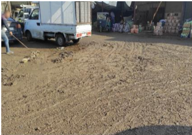
Figure 19 – Souk Al-Hal, the bad infrastructure of the market
