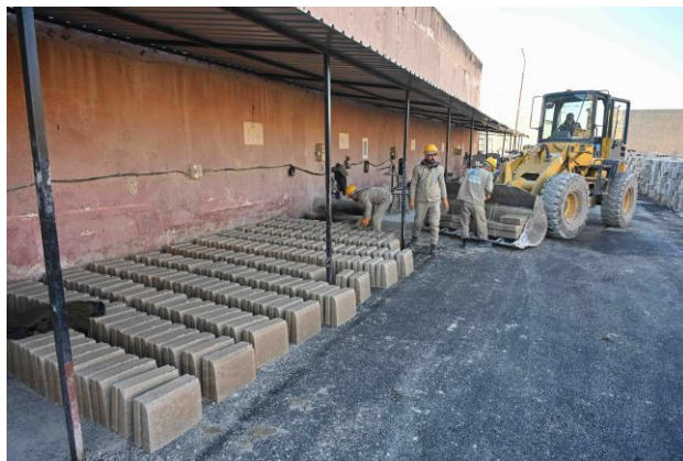
Figure 3- Debris recycling site in Al Ramoseh- Aleppo
