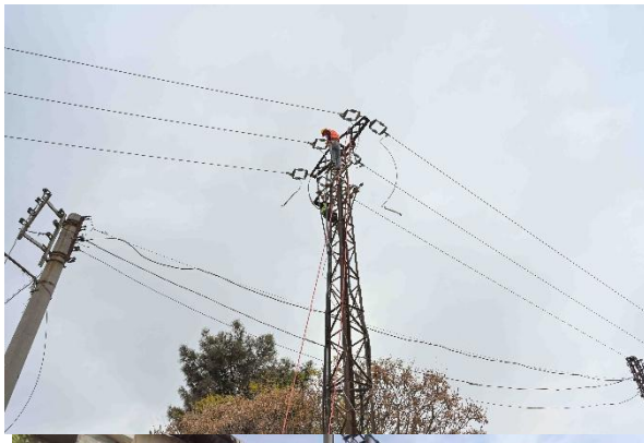
Figure 1- Electricity grid rehabilitation in Qadi Askar
