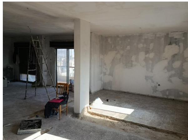
Figure 11 UN-Habitat - Rehabilitation works of the GOLD offices.
