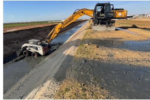
Figure 19- Cleaning of the open irrigation canal.
