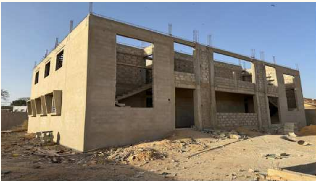
Construction of a daycare facility for the Senegal National Police, Thiès, Senegal, December 2025.
