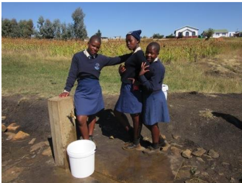
The new water system now delivers clean water from a mountain spring directly to the school grounds. Photo: UNICEF Lesotho/Ekanem
