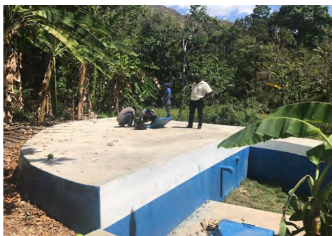
© UNDP Haiti - Construction drinking water supply system Sarazin
