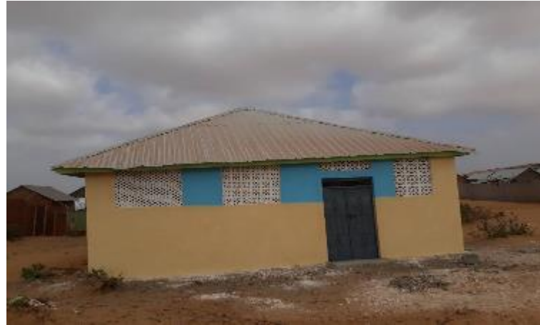
Completed market shed in Kismayo District © Omar Salad Mohamed/ UN Migration Agency (IOM) 2017
