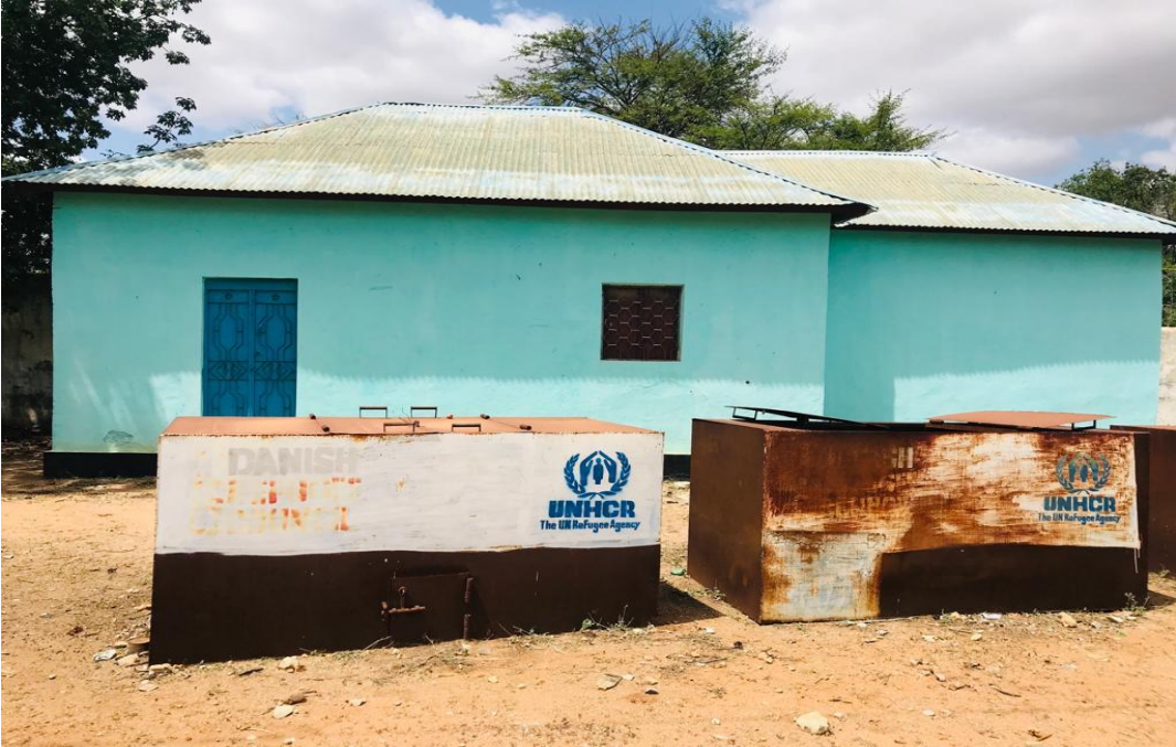
Figure 2 - Existing building to demolish and cart away debris from the site
