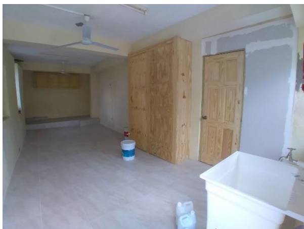
Activity Room at Cedars Home for Abused Women and their Children retrofitted by replacing carpet with tiles, and installing storage cupboards, a large sink, and a toilet facility.
