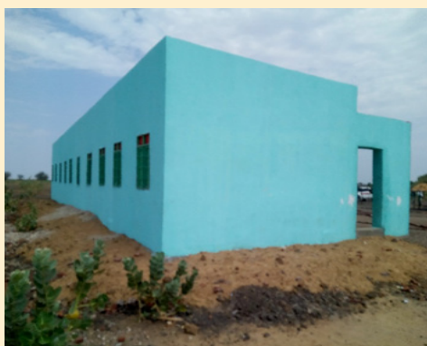
New classroom block at Jorot Primary School. Credit: ADRA
