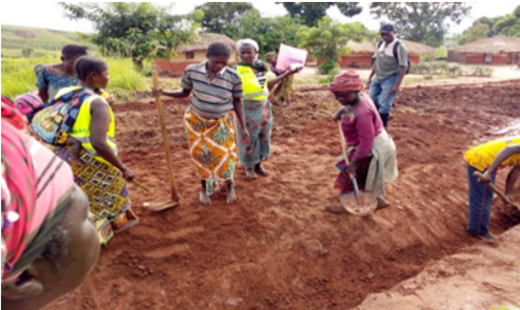
Construction of 12 km of agricultural road, PROVAH, Kalemie, Tanganyika
