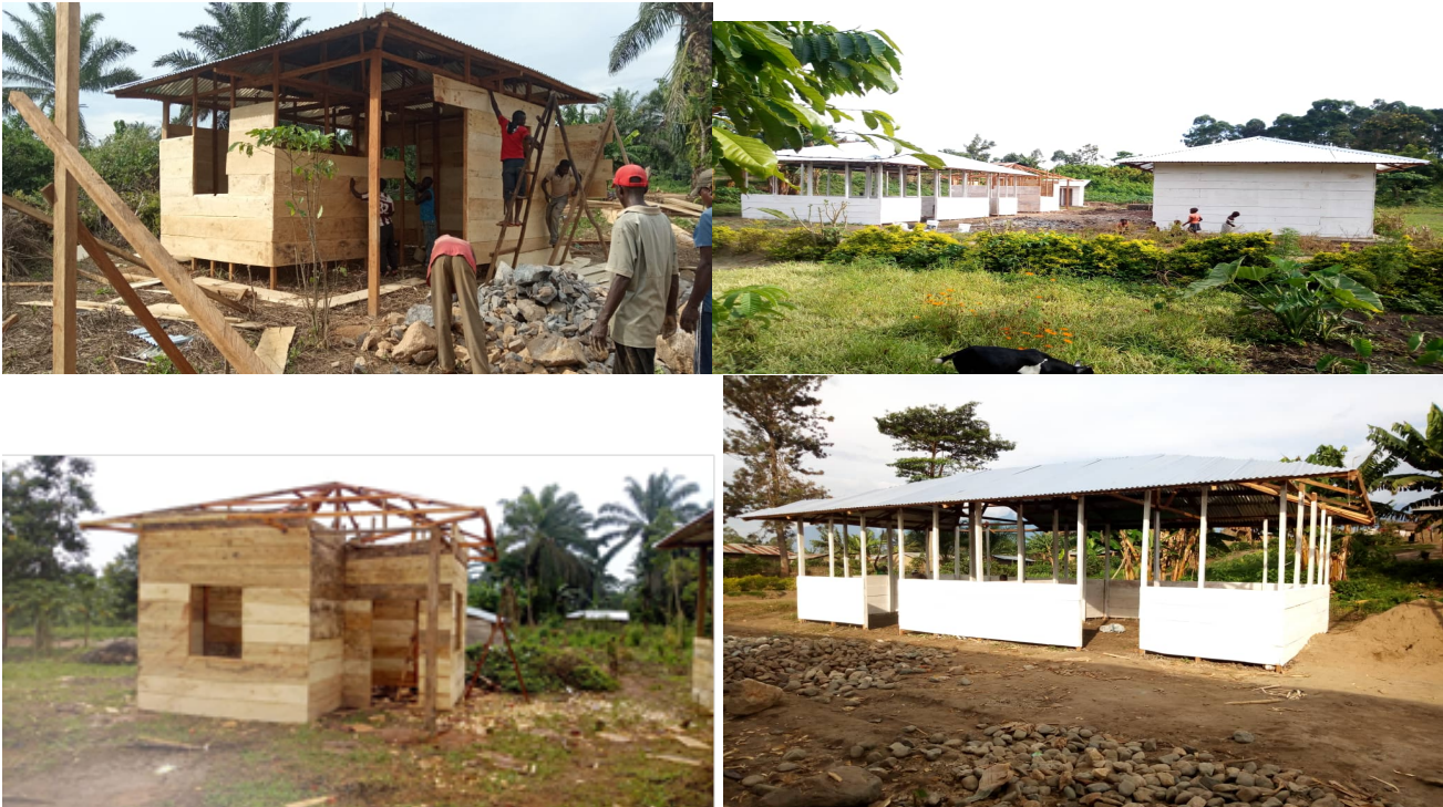
Construction of women's resource centers, CEFIDI, Beni, South Kivu
