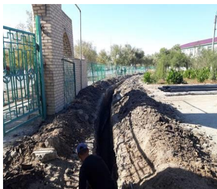
Photos 28, 29: Drinking water pipeline laying in Kungrad District Hospital
