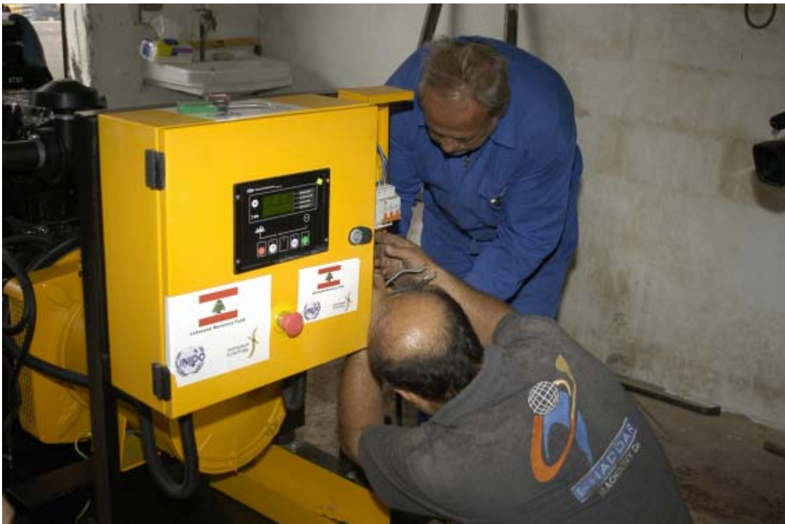
Provision of new generator, Abou Ghida, Khiam
