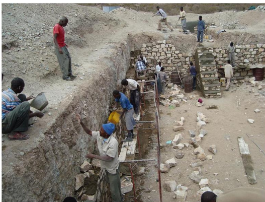
Construction of Berked (water storage) – Gurayacawl (Borama District): Construction of side walls and roof fixing.
