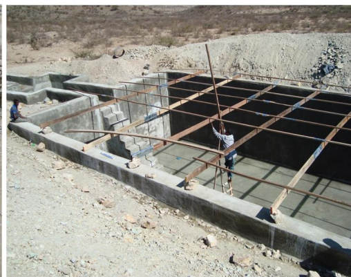
Construction of Berked (water storage) – Gurayacawl (Borama District): Construction of side walls and roof fixing.
