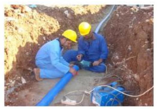
Laborers Jointing the PE Pipes Using Electrofusin Technology
