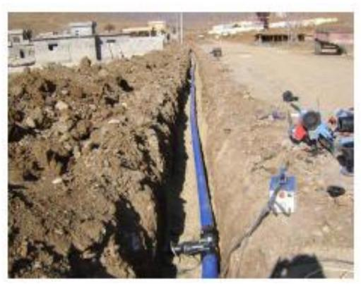
Jointing of PE Pipes using Electrofusion Jointing Technology
