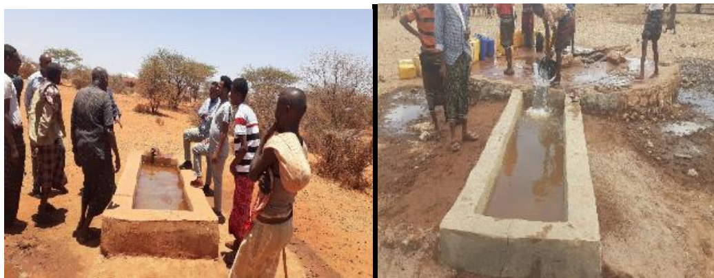
Cattle troughs constructed in Warder Woreda
