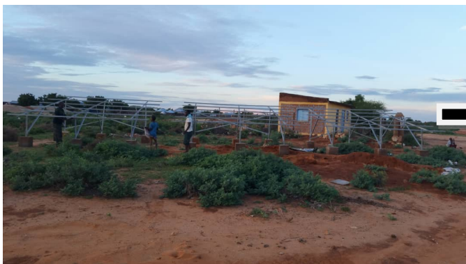
Baliwanaag Borehole rehabilitation through installing solar grids.
