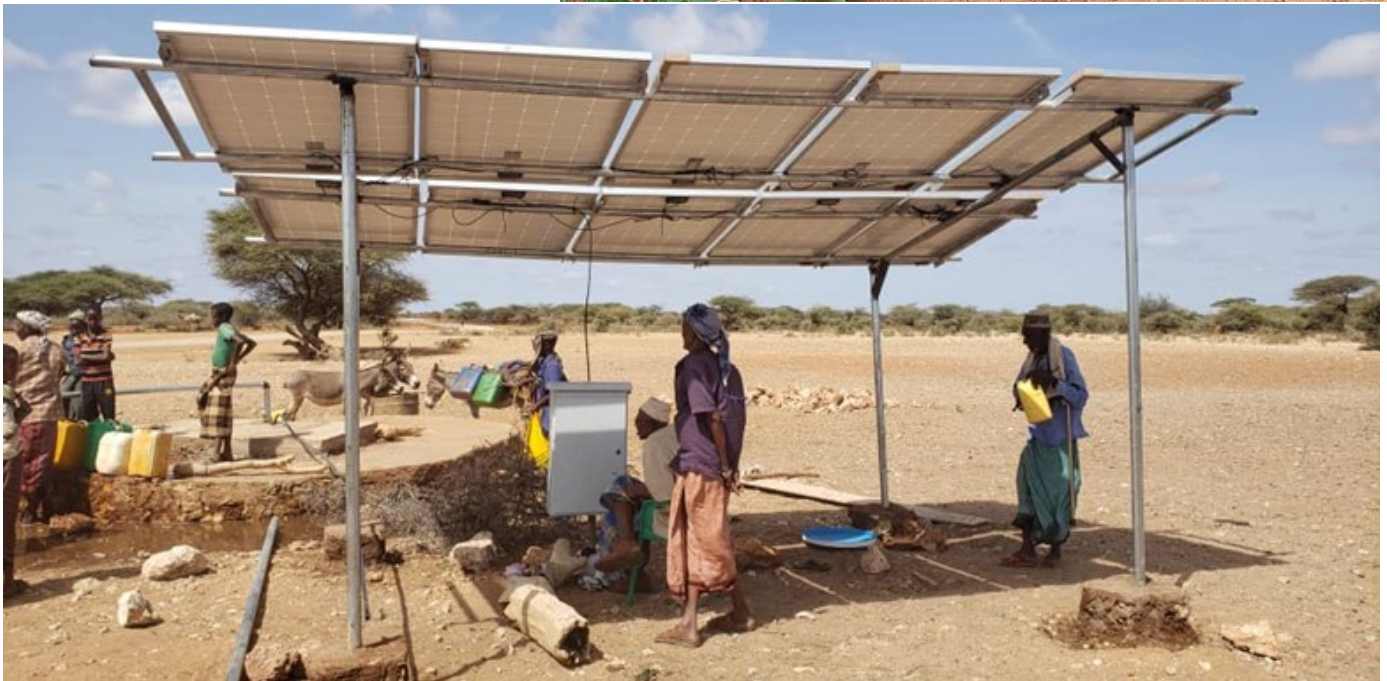
Photo 3: Left is solar water pump and Right is watermelon garden irrigated by water from the solar water pump
