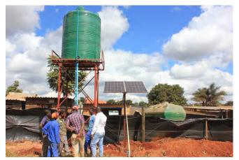
Installation of a tank, solar panel and tap at the Hatcliffe market will ensure an uninterrupted supply of water and improve hygiene for vendors and the local community. © Helpline Zimbabwe
